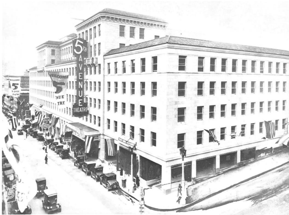
Fig.15 The Skinner Building, containing the 5 th Avenue Theatre, facing northwest, 1926 (Terry Helgesen Collection)
